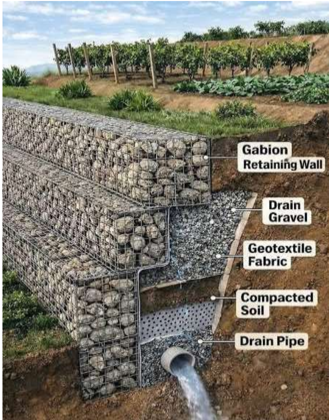
Figure 2: Gabion Retaining Wall as an Erosion Control Measure, Bida LGA.
